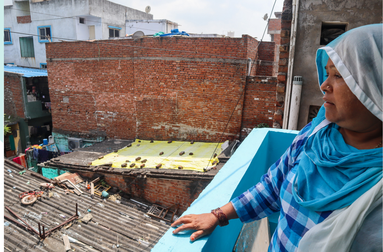
From the balcony of her first-floor bedroom, Hazra Banu shows me the neighbouring houses to illustrate what her house looked like a year ago. Ahmedabad (September 2019)
